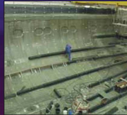
Rib formers for FRP marine construction.
